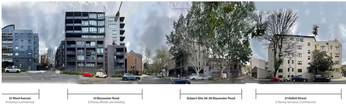
Figure 2: Existing streetscape along Ward Avenue (Source: Design Report, Squillace Architecture + Interiors)
